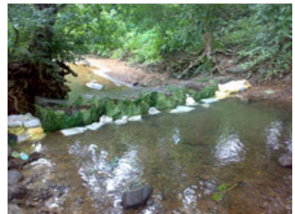
The Alaknanda group built a rooftop water-harvesting system (top) for a local school during Water RYLA 22-24 August, in villages of Kelva Beach, Palghar, India. (Bottom) The Ravi group completes a reservoir dam. Photo courtesy of Water RYLA
