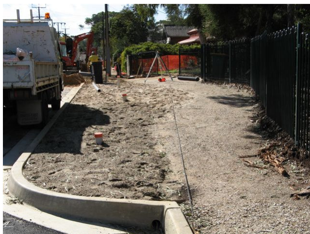
Under verge water storage works in progress in George Street.
