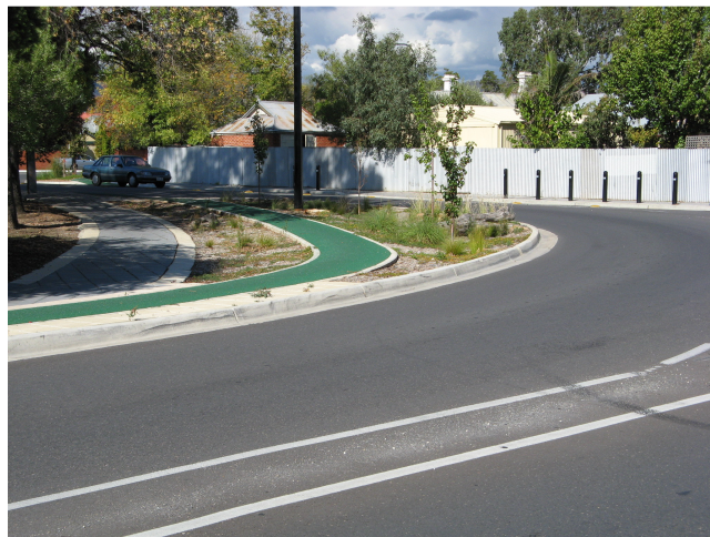
A completed section of the George Street/Maud Street road works.
