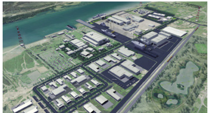
The new "Techport" under construction at Osborne
