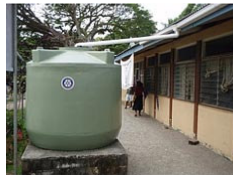
Water tank at a Solomon Islands school
