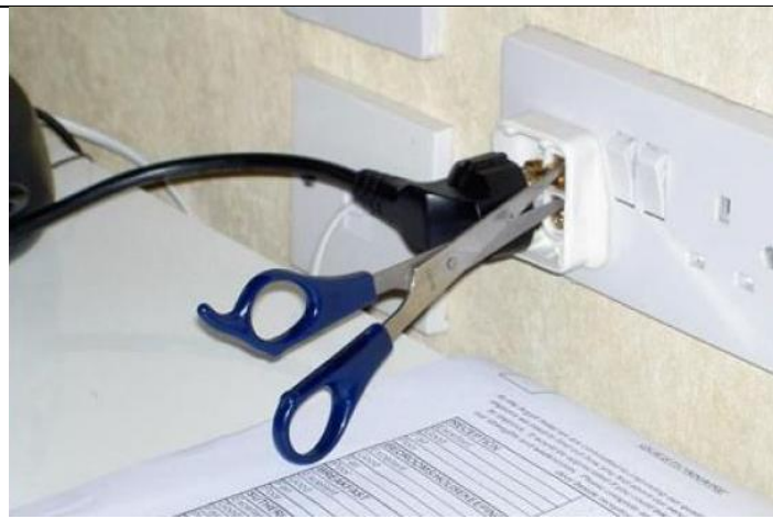
Fixing the electricals
