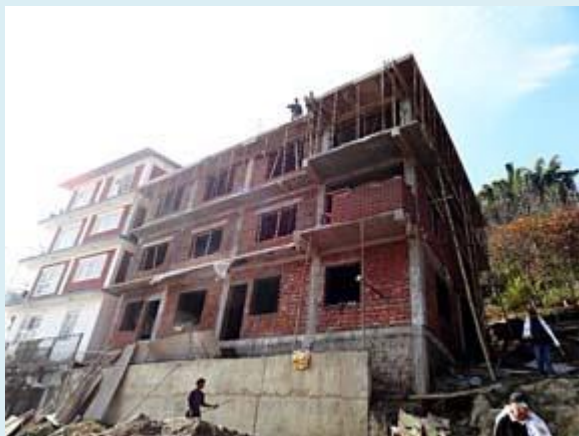
Full steam ahead with the DMUK orphanage on the left and the school on the right. This photo was taken in late December. The February deadline will be tight!
